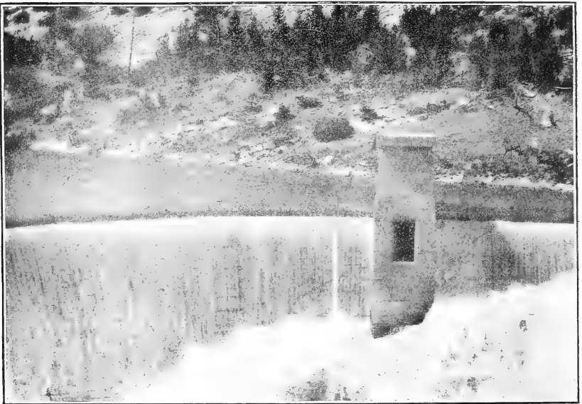
FIG. 2.—ARCHED TYPE SPILLWAY DAM, PISHKUN RESERVOIR, MONTANA. Air intake tower shown in center of picture built to eliminate vibration due to vacuum.
